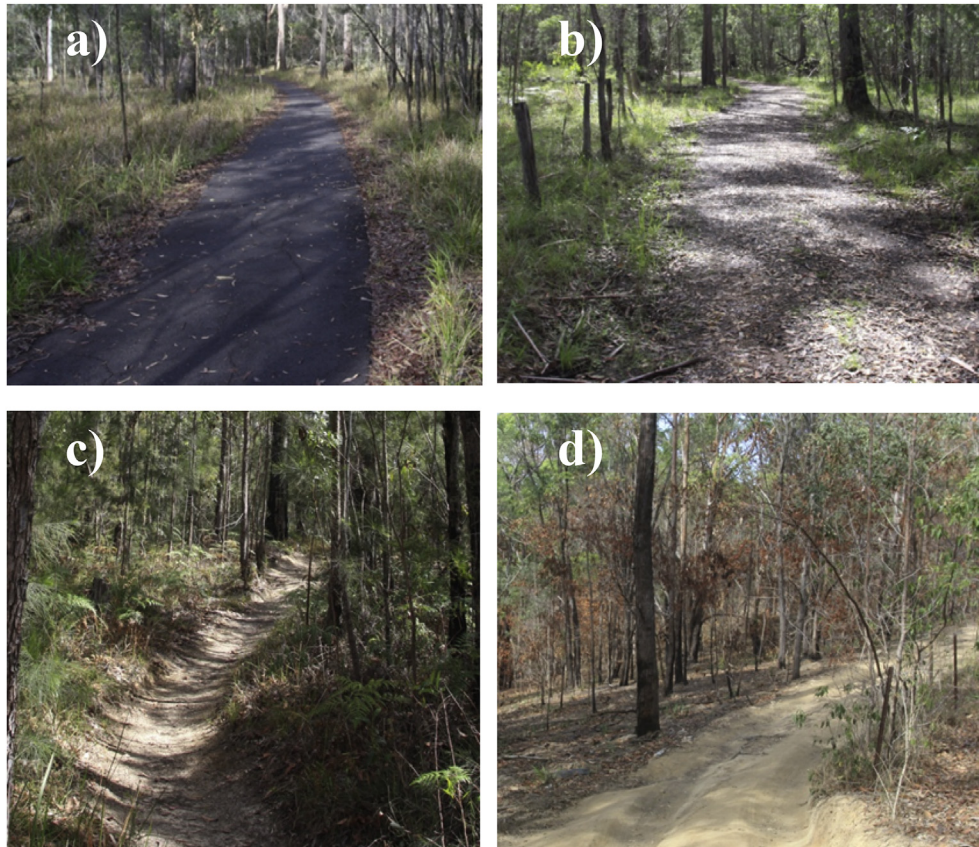
Fig. 2. The four trail types assessed (a) tarmac/concrete (2–4 m wide) and (b) gravel (2–4 m wide) formal trails, and (c) narrow (<2 m wide), and (d) medium width (2–4 m wide) informal bare earth trails.
